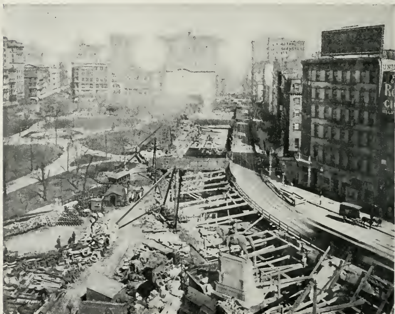
Subway Construction at Union Square and Fourth Avenue.
